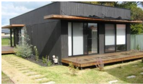
Unit Unit 2, 20 Wattletree Grove, Benalla
