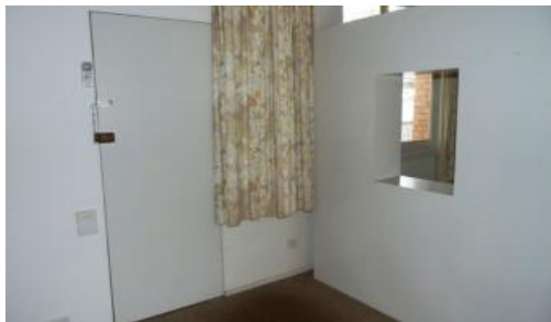
Unit 6, 34 Bridge Street, Benalla
